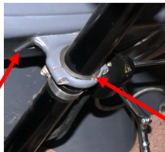
Tank can weep here.
