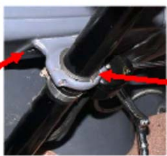
Tank can weep here.
