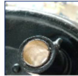
New bushings installed.
